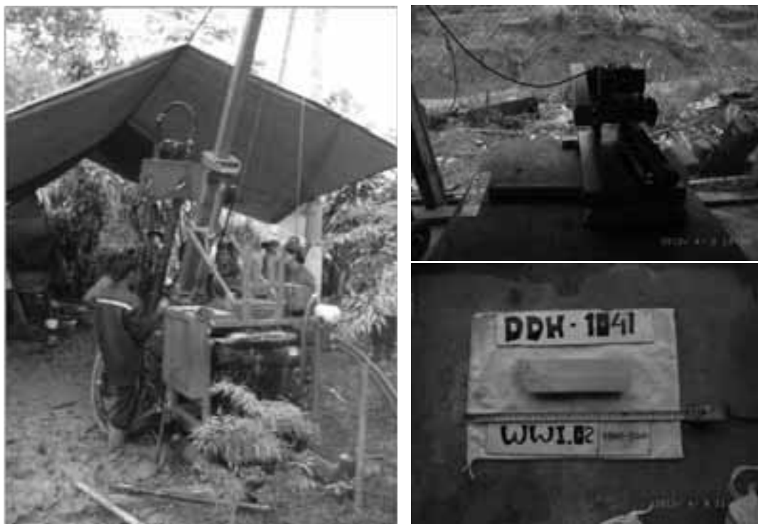
a: working drill rig at Cikadu
